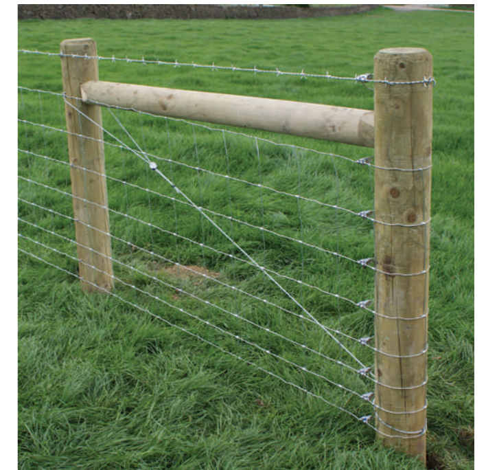
GPAK 3 - Bracing the end of a fencing run.
